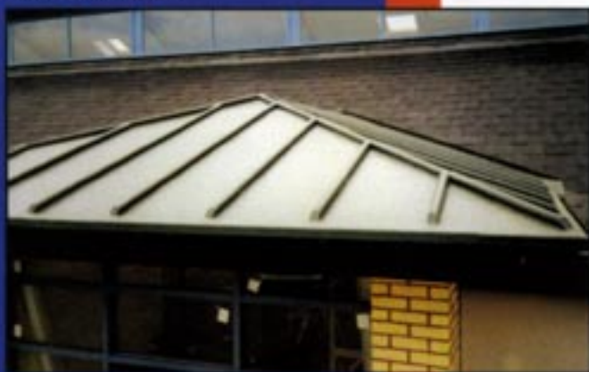
Below: Lead roll is not just suited to older properties as this new building below illustrates.
